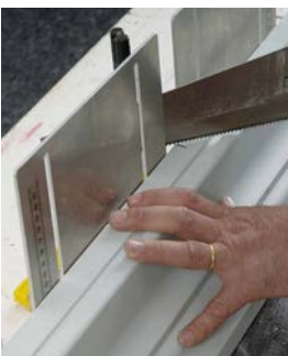
WINDOW SILL PROFILE ANGLED ON BOTH SIDES
