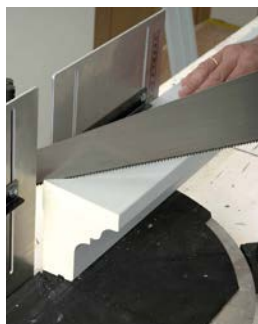
WINDOW SILL PROFILE ANGLED ON BOTH SIDES
